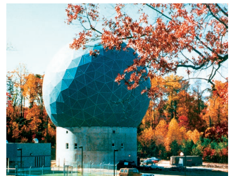
100 ft. (30.6m)-diameter MSF radome.
