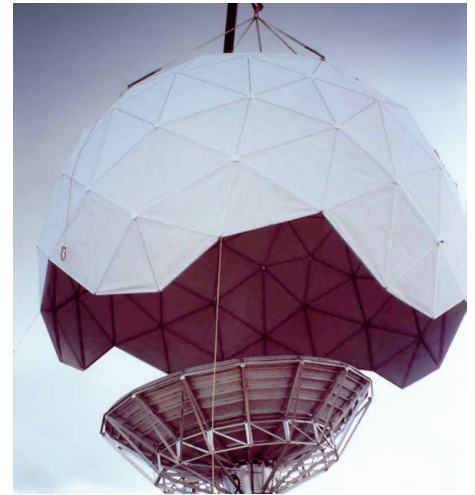
Typical 48 ft. (14.7m)-diameter MSF radome installation.
